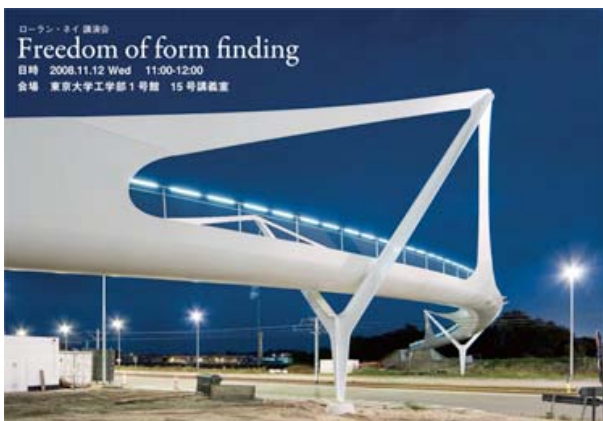
写真-3 Footbridge Knokke-Heist
